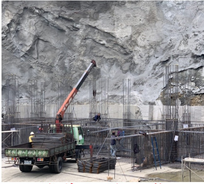
筏基鋼筋綁紮
